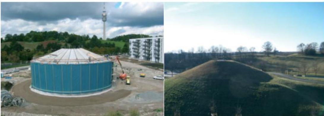
**Fig. 10.5 Large Hot water storage (construction and final state) [33]**
