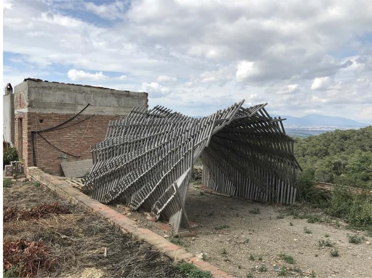
**Obrázek 1.1:** The entire shelter was assembled by 6-axis robotic arm, which also formatted each individual wooden beam (Masia Can Valldaura, Barcelona, Spain). Photographed by the author in 2018.
