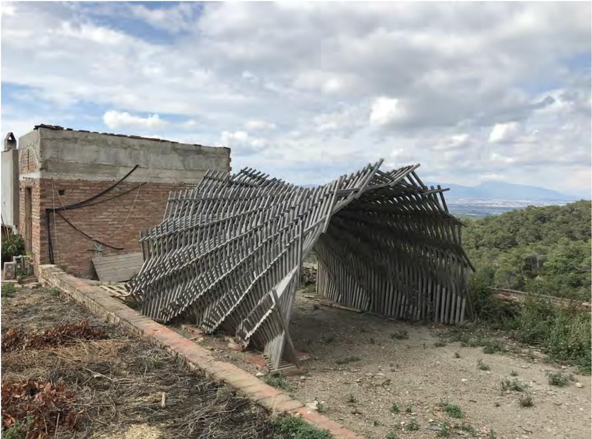
**Figure 2.1:** The entire shelter was assembled by 6-axis robotic arm, which also formatted each individual wooden beam (Masia Can Valldaura, Barcelona, Spain). Photographed by the author in 2018.
